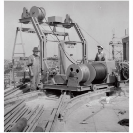
Window cleaning hoist, Sydney CBD. 1960's
