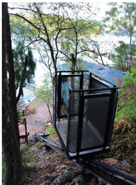
Half-cab with curved edges and perforated aluminium side infill panels in colour black
