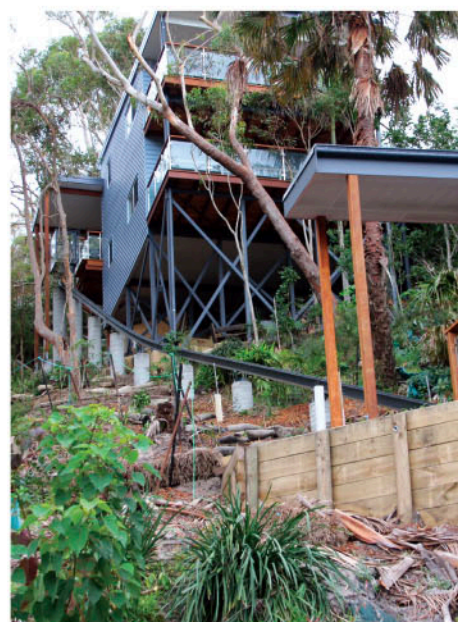
Change in rail gradient available to a maximum of 8 degrees over total length of travel
