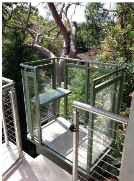
Half-cab with folding seat, curved edges in colour mist green with clear acrylic side infill panels
