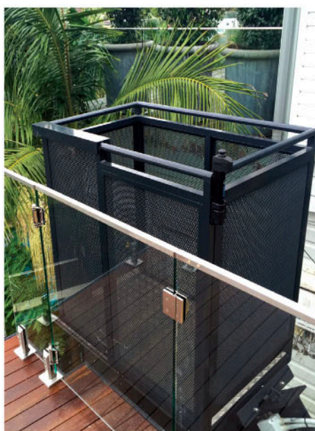
Half-cab with electrically interlocked manual sliding door and perforated aluminium side infill panels in colour charcoal
